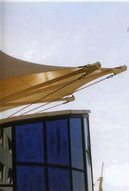
A threaded adjusting device elongates the catenary cables and provides tension for the canopy.
