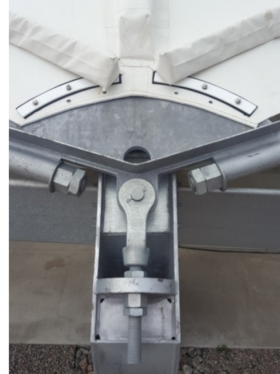
Figure 10: Typical "floating" membrane plate
