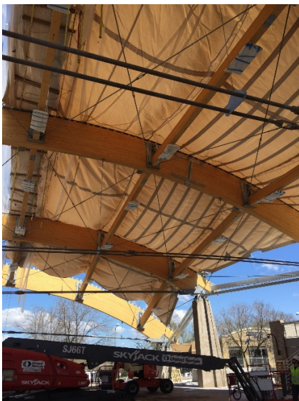
Figure 11: Fabric reinforcements during erection
