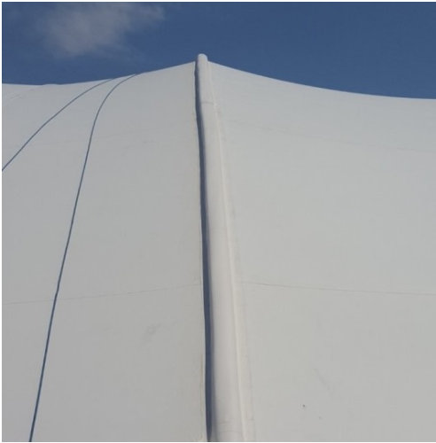
Figure 13: Fabric closure at arch top
