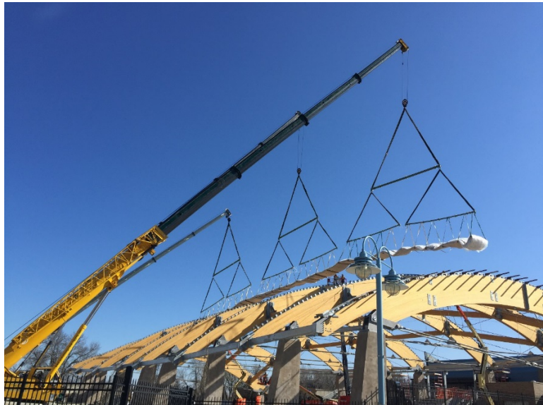
Figure 12: Three cranes with spreader bars placing fabric
