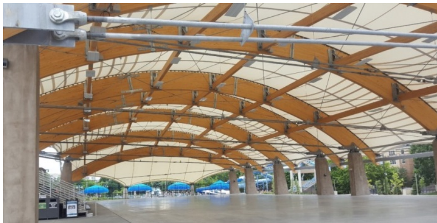
Figure 3: Interior view, looking south, showing glu-lam arches, fabric reinforcement
