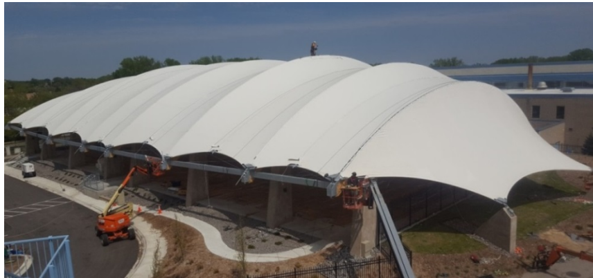
Figure 2: The roof structure nearing completion
