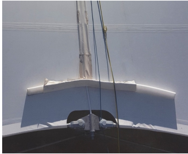
Figure 14: Valley closure / diverter intersection
