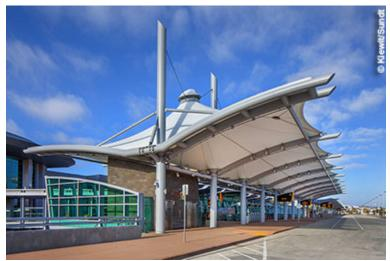
The new outdoor ticket counter pavilions at San Diego International Airport are capped by large fiberglass canopies that cantilever on two sides and are supported by suspension cables. © Kiewit/Sundt
