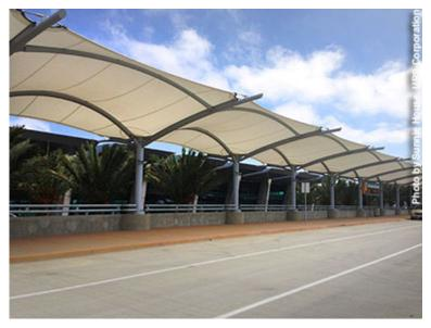
The canopies atop the new elevated deck roadway at San Diego International Airport were fabricated with Teflon-coated fiberglass, which is strong and durable as well as translucent. Photo by Sunnie House, URS Corporation
