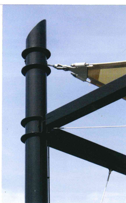
Vertical cross bracing with steel cables maintains a visually light appearance.
