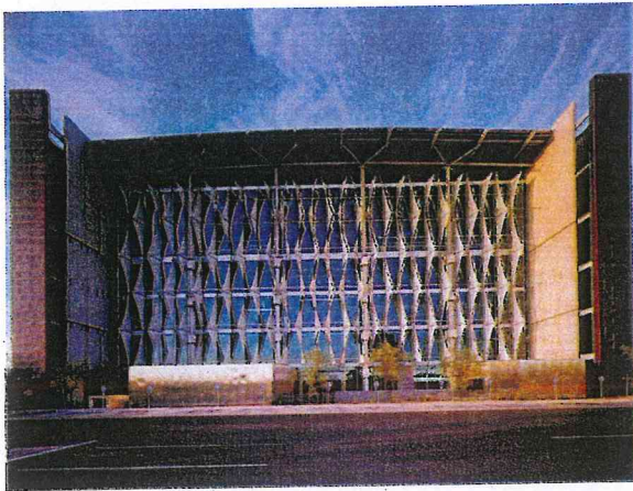
Figure 18.9 The vertical fabric mesh sunshades at the Phoenix Central Library provide dramatically different effects, depending on ambient lighting conditions. They appear nearly opaque in daylight, but have gossamer transparency at night.
