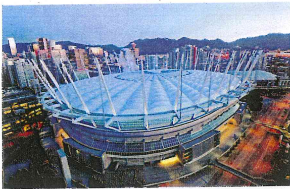
Figure 18.16 The BC Place Stadium renovation included the installation of a new roof with radiating overhead and underslung cables that support the fabric roof. The grandstand covers are fixed fabric panels, while the center section employs retractable TENARA pneumatic cushions.
