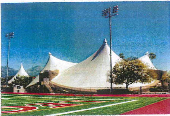
Figure 18.2 The University of La Verne Campus Center, completed in 1973, made the first use of the new PTFE-coated fiberglass fabric. Its original membrane is still in service today, with only modest loss in fabric strip tensile strength.
