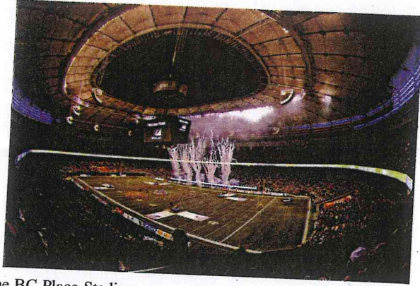
Figure 18.17 The BC Place Stadium renovation included the installation of a new roof with radiating overhead and underslung cables that support the fabric roof. The grandstand covers are fixed fabric panels, while the center section employs retractable TENARA pneumatic cushions.
