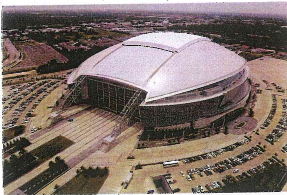
Figure 18.14 The translating center section of the Cowboys Stadium roof demonstrates the use of fabric in a versatile retractable-roof application, though the fabric functions more as cladding than a spanning element on the synclastic “skylight” form.
