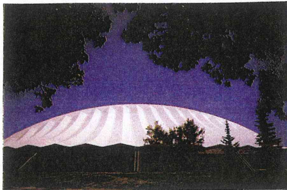
Figure 18.4 Talisman Centre in Calgary, Alberta, was reroofed using an aerogel fabric that provides effective insulation while maintaining significant translucency.
