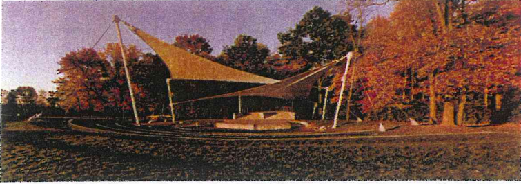
Figure 18.5 The amphitheater in Springboro, Ohio, uses minimally curved membranes to dramatic effect, while employing heat trace cables and drainage openings in the lower membrane to address extreme weather events.
