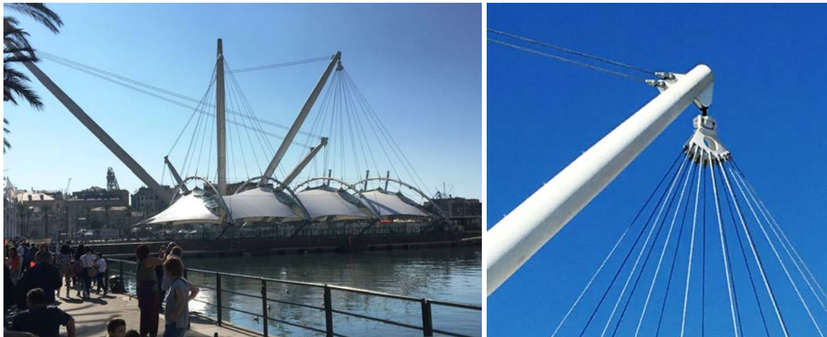
Figure 5. Bigo's structural elements are all exposed, and clearly display the load path.
