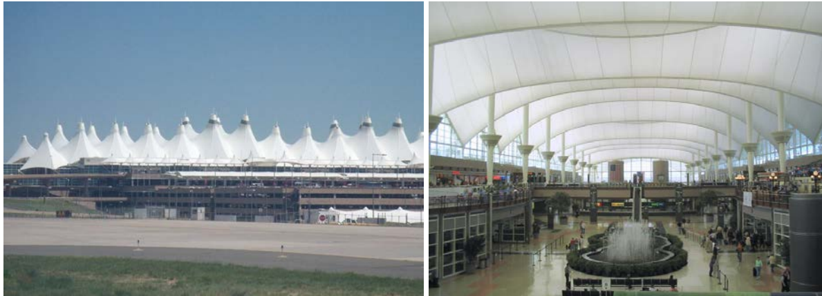
Figure 3. The Denver Airport Terminal's roof design pursued lightness and efficiency, with beauty the result.
