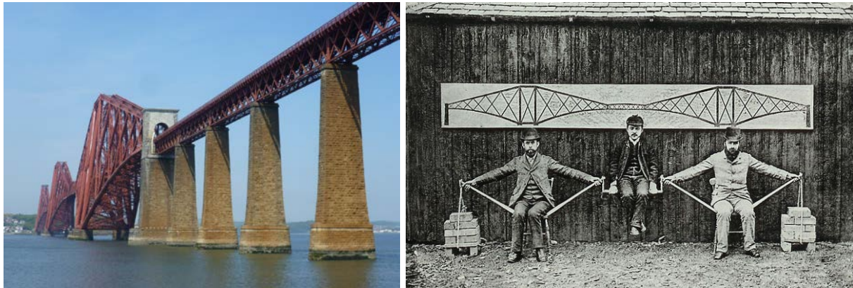
Figure 6. Human “members” were used to model the load-bearing action of the Firth of Forth railroad bridge.
